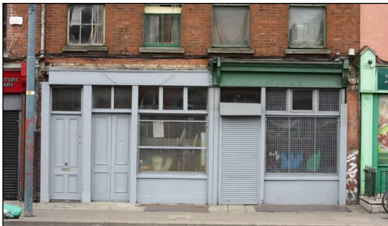
Figure 3: Detail of two shopfronts on ground floor front elevation
