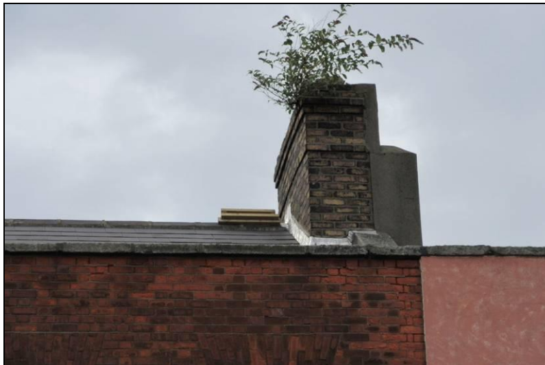
Figure 10: Yellowbrick chimneystack on northeast end of roof
