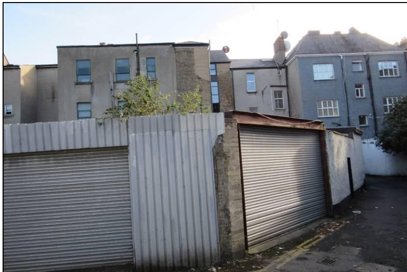
Figure 13: View of rear elevation and rear lane
