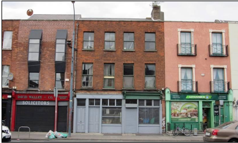
Figure 2: 55 Amiens Street in terrace of buildings
