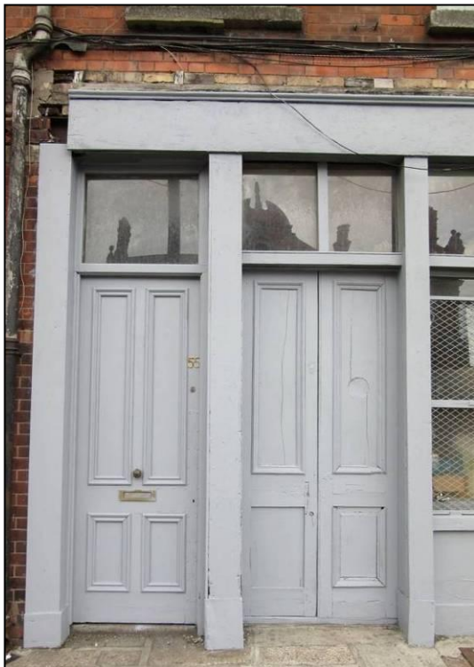
Figure 4: Detail of doors on front elevation of building
