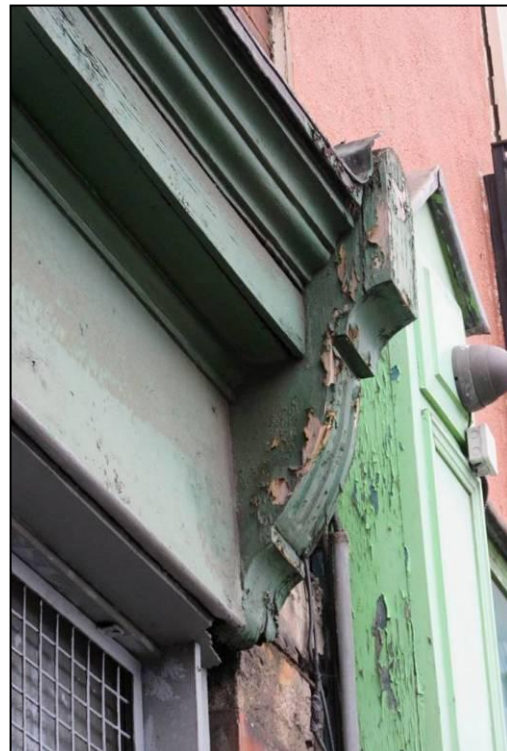
Figure 5: Detail of consile bracket on shopfront
