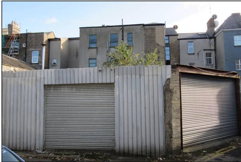
Figure 12: View of rear elevation and rear site of structure
