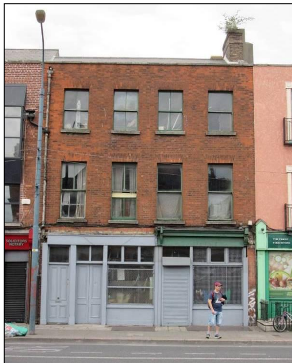
Figure 1: Front elevation of 55 Amiens Street
